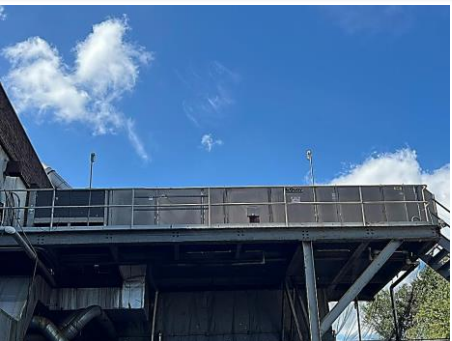
View of 300 Ton Chiller
